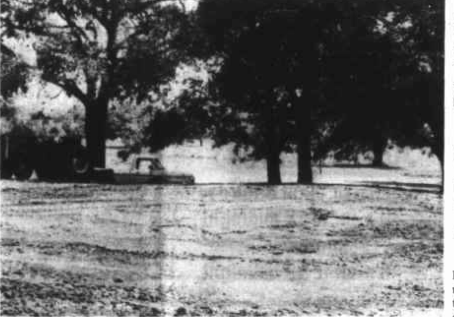
Golf greens under repair The Recreation Center golf course is undergoing repairs and will remain closed for about two months. The common bermuda grass used on the greens is being replaced by a new Tif variety that will enhance playability.
